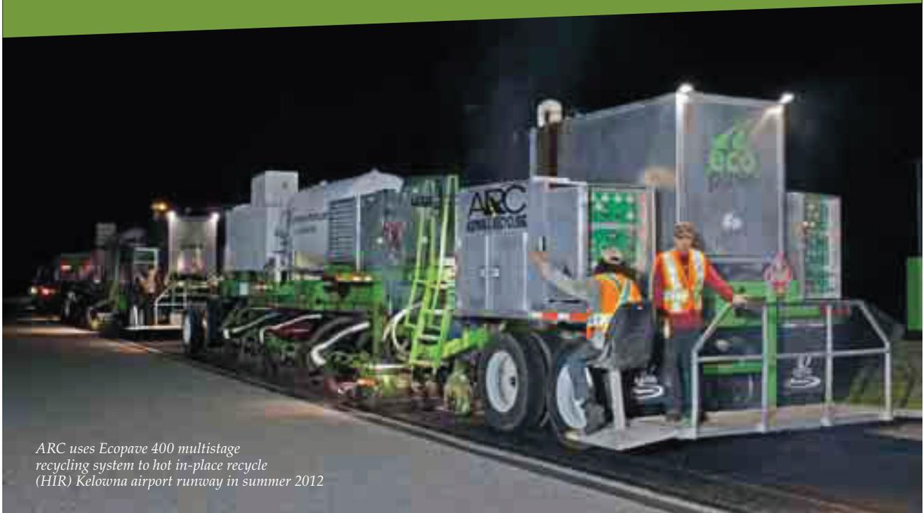
*ARC uses Ecopave 400 multistage recycling system to hot in-place recycle (HIR) Kelowna airport runway in summer 2012*
