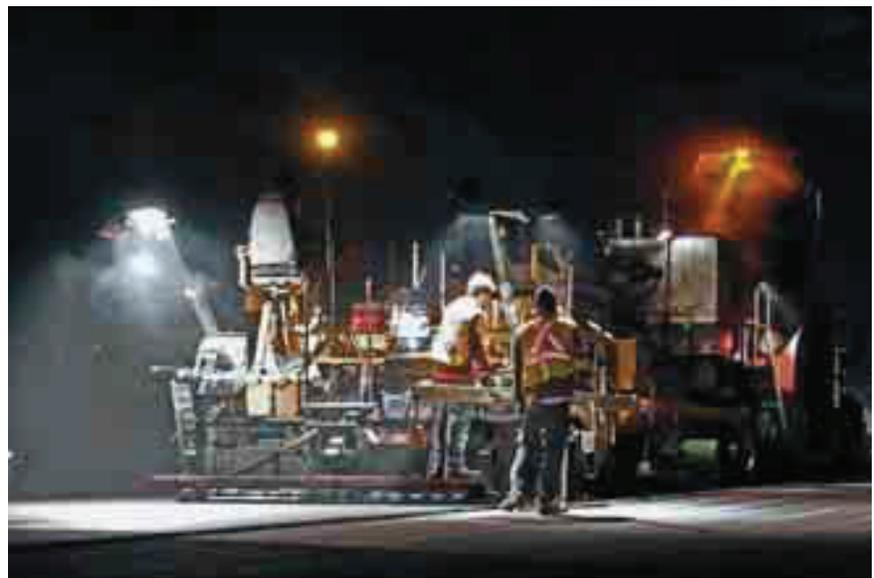
At Kelowna airport HIR project, recycled asphalt mixture is placed by a Cat AP 1050B paver
