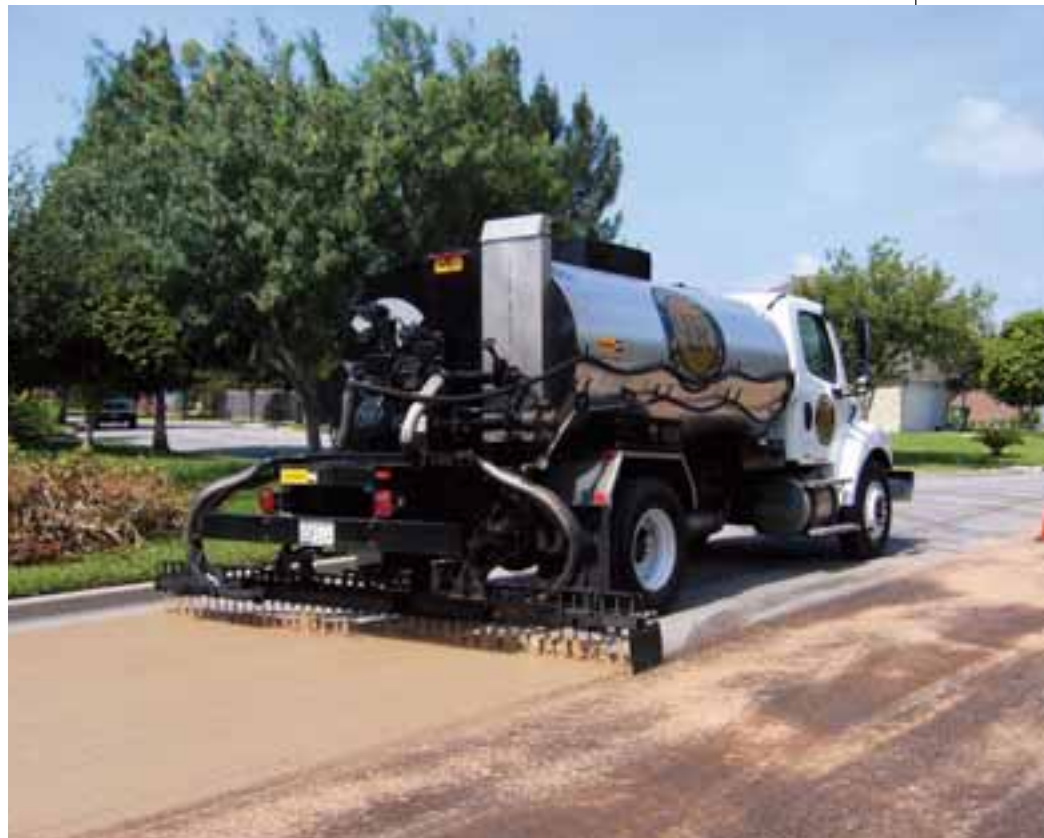
Pavement Restoration, Inc., Boerne, Tex., applies Reclamite rejuvenator to pavement in Travis County, Tex.
